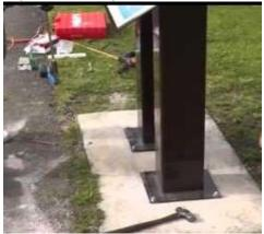
frame. Renovation and rehabilitation of existing masonry structures usually require that anchor bolts be used to attach stair risers, elevator tracks and various frame assemblages for equipment installation.
